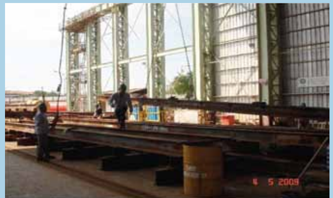
Fabrication of tables for WPG
