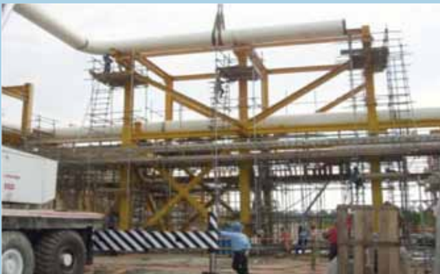
Piping activities at main pipe rack
