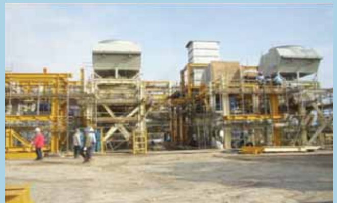
Activities at turbo compressor area : lube oil TBC A erected
