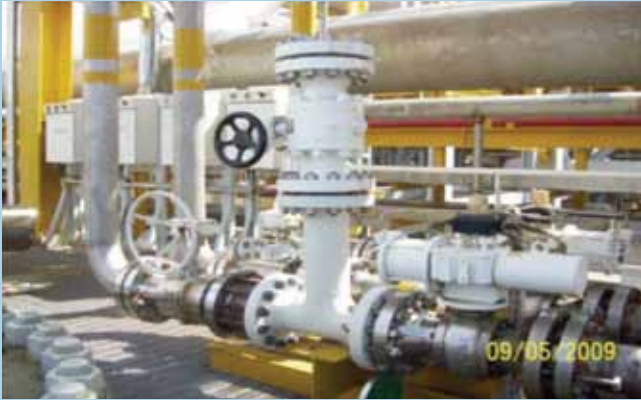
Completed tie-in G20
