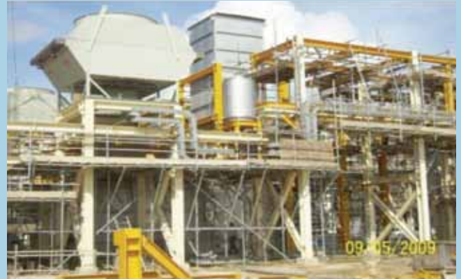
Completed demister installed at turbo compressor B & A
