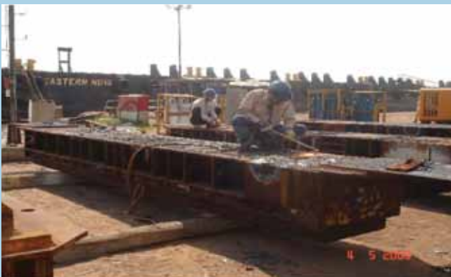
Fabrication of cross beams & skid shoes
