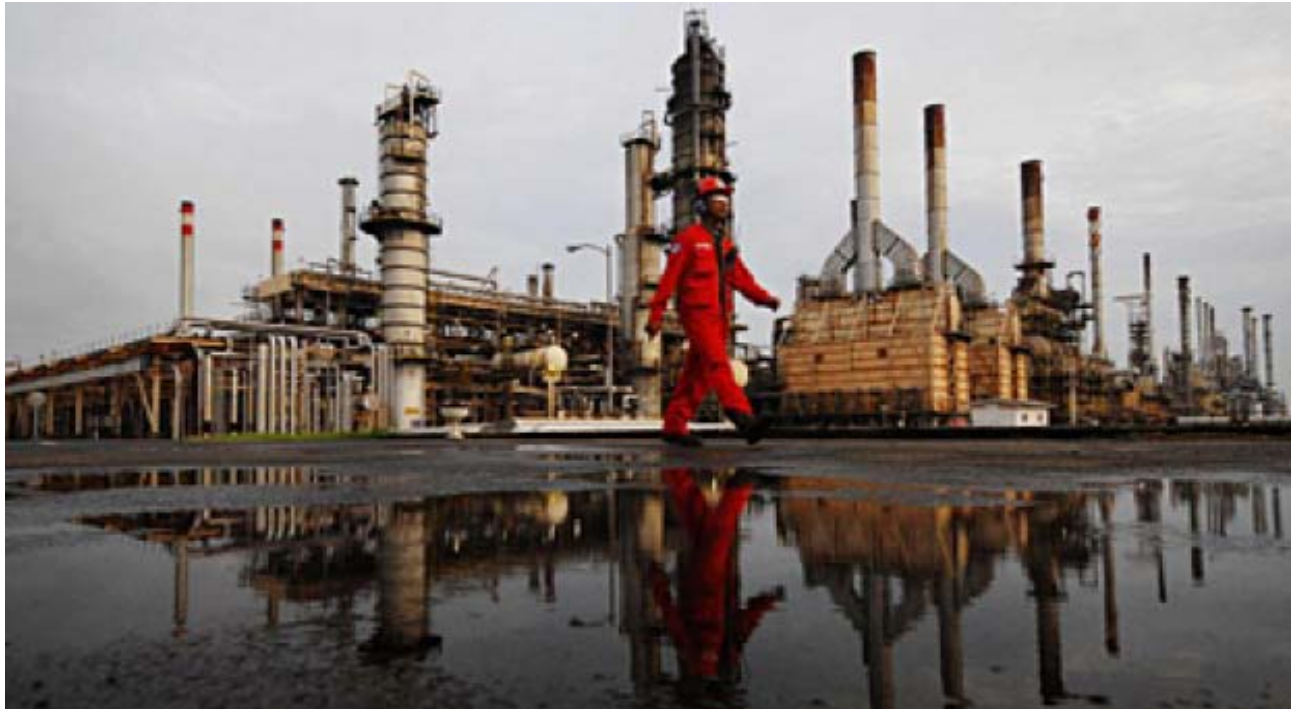
Fuel Oil Complex 1 di Kilang Minyak Pertamina Refinery Unit (RU) IV, Cilacap, Jawa Tengah. TEMPO/Panca Syurkani
