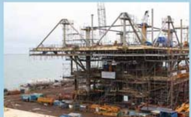
CPP Deck Erection
