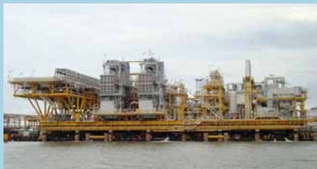
South Compression Platform (SCP)
