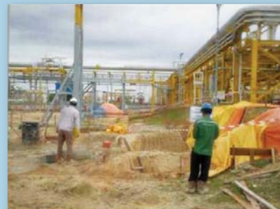
Main Pipe Rack Foundation
