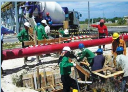
Concrete Pouring for Sensitive Wells Foundation Started on May 24, 2008
